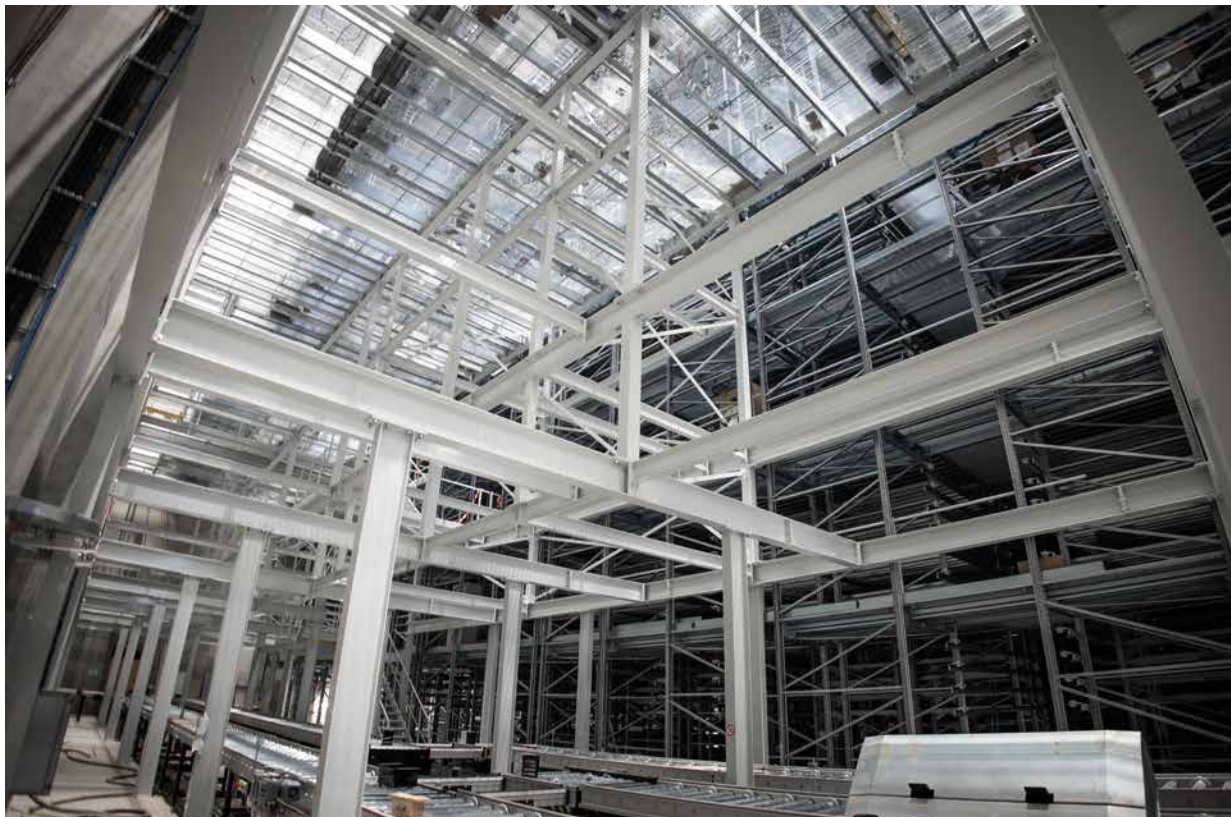
Custom platforms for large Mezzanine Structure
